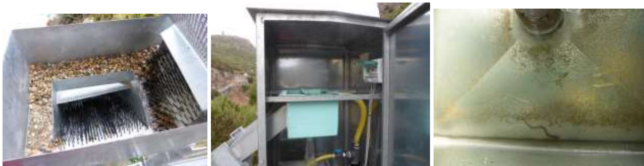
Figure 6. Details of the sluice (left), of the monitoring cabin (centre); a juvenile specimen trapped during the first monitoring phase (right).
