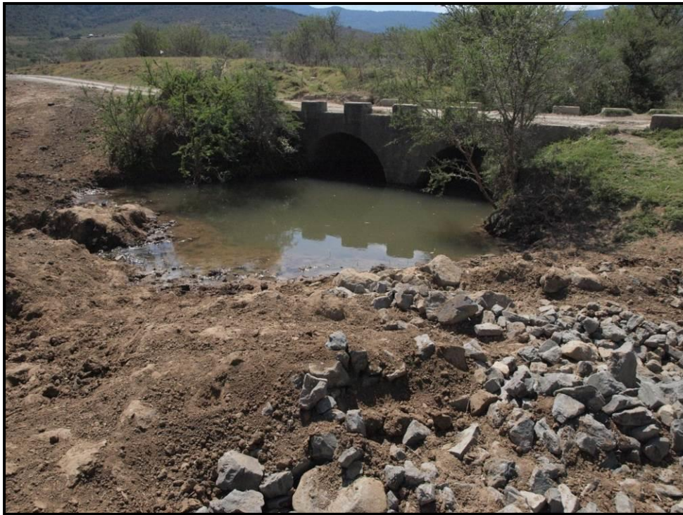
An example of a highly degraded and modified section of a Keiskamma River headwater tributary where border barbs were absent
